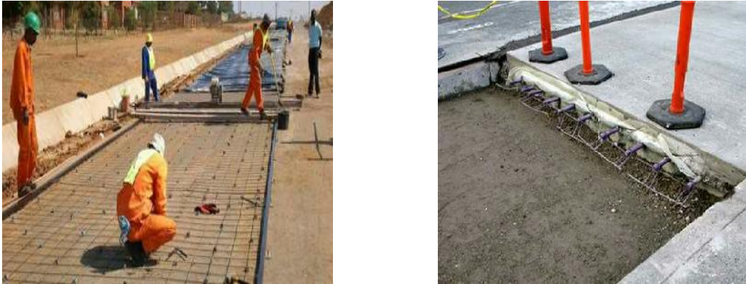
Fig. 2: Cement Roads being built by Ikpeazu in Aba (4:42pm on 9th October, 2015)
