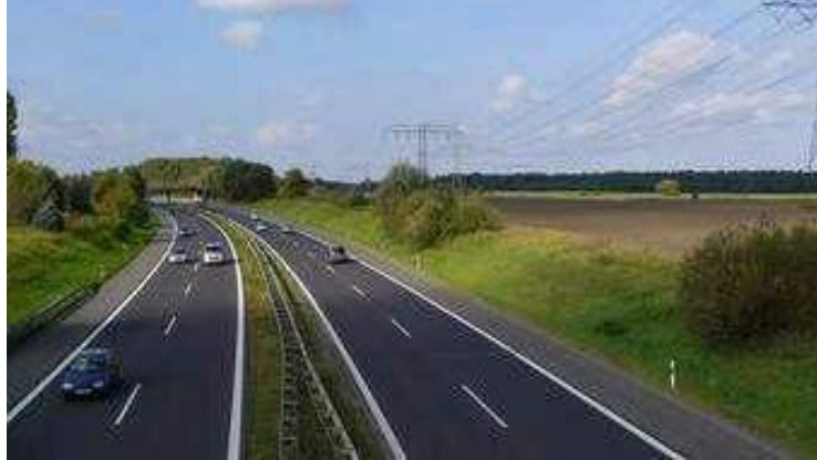
Fig. 1: The Asphaltic Roads being built by Ikpeazu in Aba (4:42pm on 9th October, 2015)
