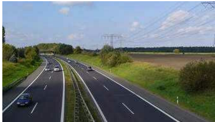
Fig. 1: The Asphaltic Roads being built by Ikepeazu in Aba (4:42pm on 9th October, 2015)
