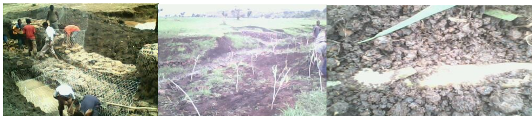
Fig. 4: Gabion check dam construction and planted branch cuttings by direct and layering on reshaped gully
