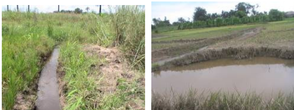
Figure 2: Constructed canal from the spring source and the artificial pond for supplemental irrigation.
