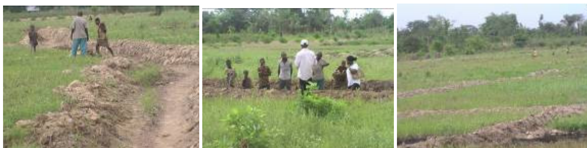
Figures 3: Construction of interceptive canals and bund making for sawah field development
