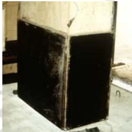
Fig. 2. Steel jacketing of a column [7].
