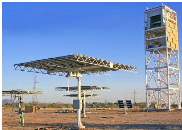
Fig. 1 Experimental Thermo-Solar Plant in Sonora, México. [14]
