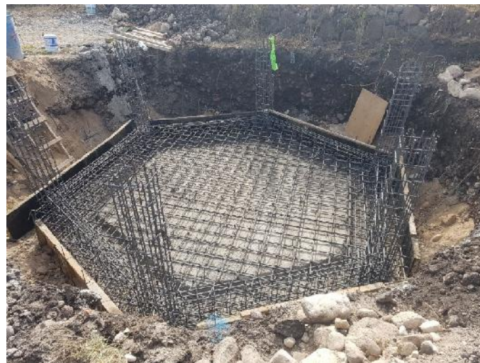
Fig. 3 Concrete Foundation of UAQ's tower
