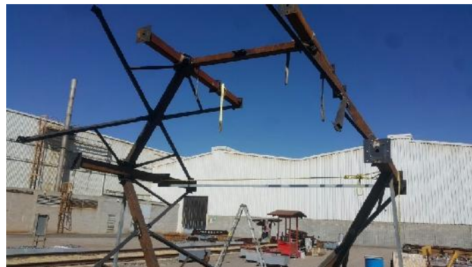
Fig. 2 Steel restricted Frames of UAQ's tower
