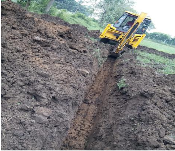
Fig.1. Installation of drain pipe
