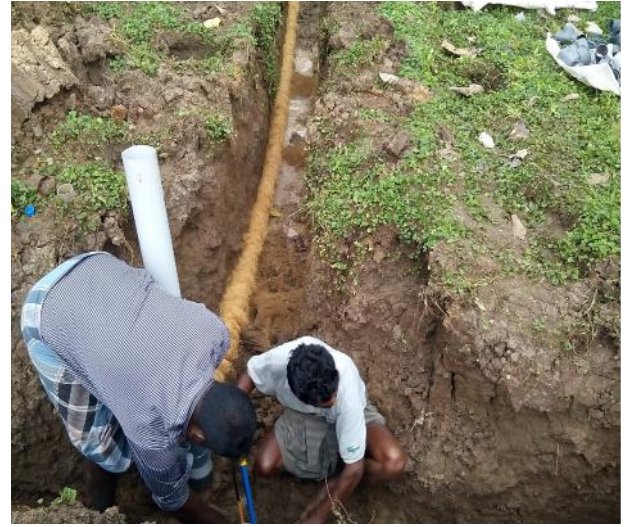
Fig.1. Installation of drain pipe
