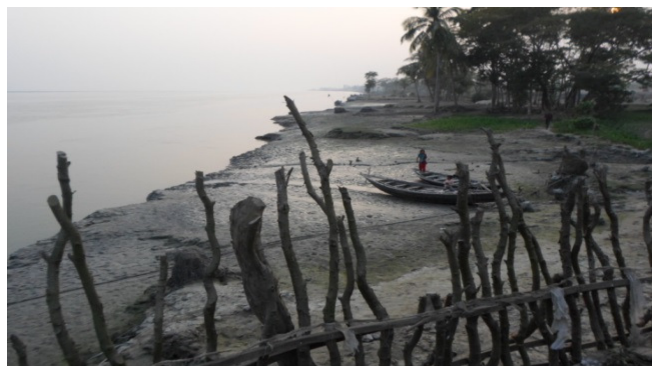
Fig.5. Photographic view of bandaling structure used for controlling bank erosion at Kajal river side in Galacipa.
