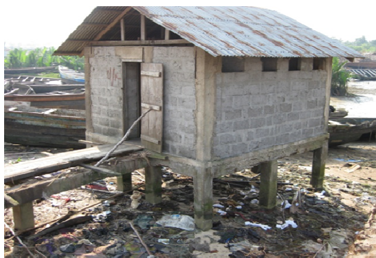
Plate 2: A typical latrine in Ibaka where deposited excreta was carried by receding tide
