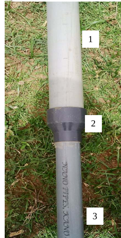
Fig. 3: The joint of a Penstock configuration
