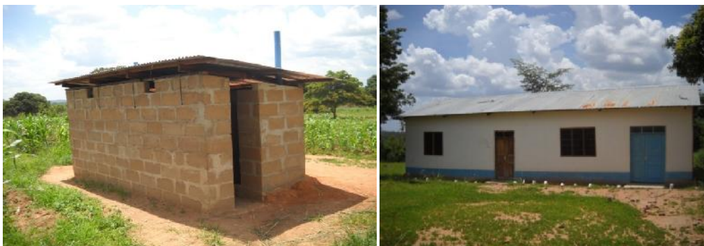
Plate 2: Pit latrine in Mwamagembe Primary School and Village Office built by support from hunting companies in Mwamagembe Villages
