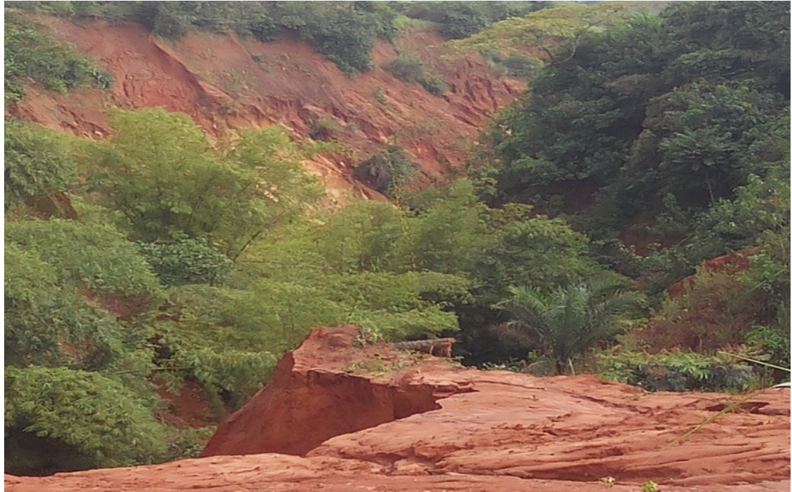
Plate 1: Severe gully site, Umueshi, Imo State, Nigeria
