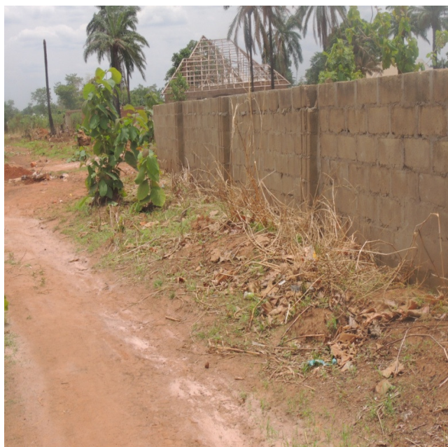
Plate 2: Opening up of roads in the reserve.
