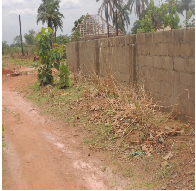
Plate 2: Opening up of roads in the reserve.
