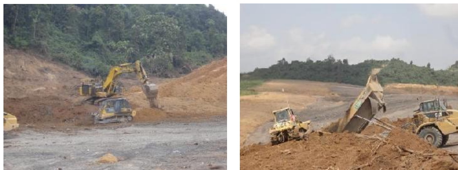
Fig. 2. Topsoil stripping and placement
