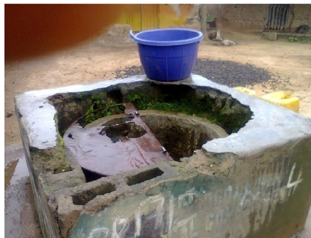
Plate 1: A hand-dug well covered with rusted iron lid at Pontela (Ogo-oluwa LGA) (Source: Author's fieldwork, 2012)
