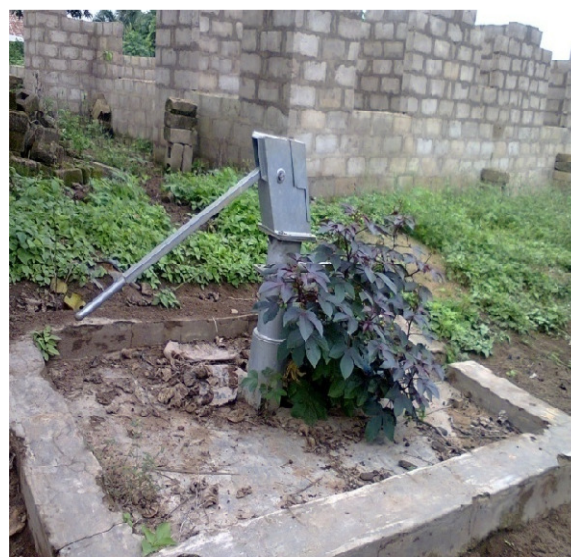
Plate 5: An Abandoned motorised borehole (due to poor water yield) at Onipanu (Surulere LGA) (Source: Author's fieldwork, 2012)
