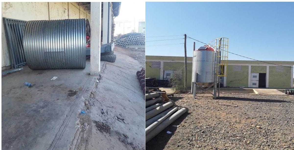
Figure: Metal silo
