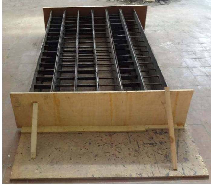
Fig. 4. Formwork in vertical position for concrete pouring.
