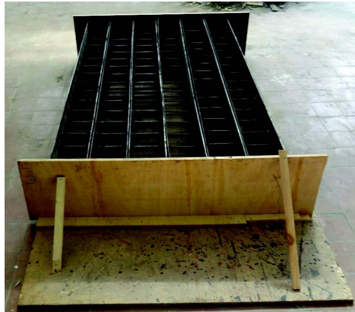
Fig. 4. Formwork in vertical position for concrete pouring.
