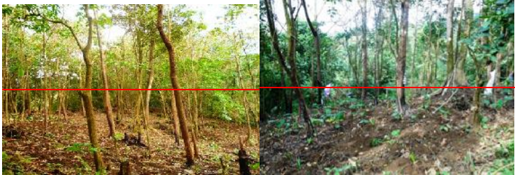
(a) Removal of the understorey
